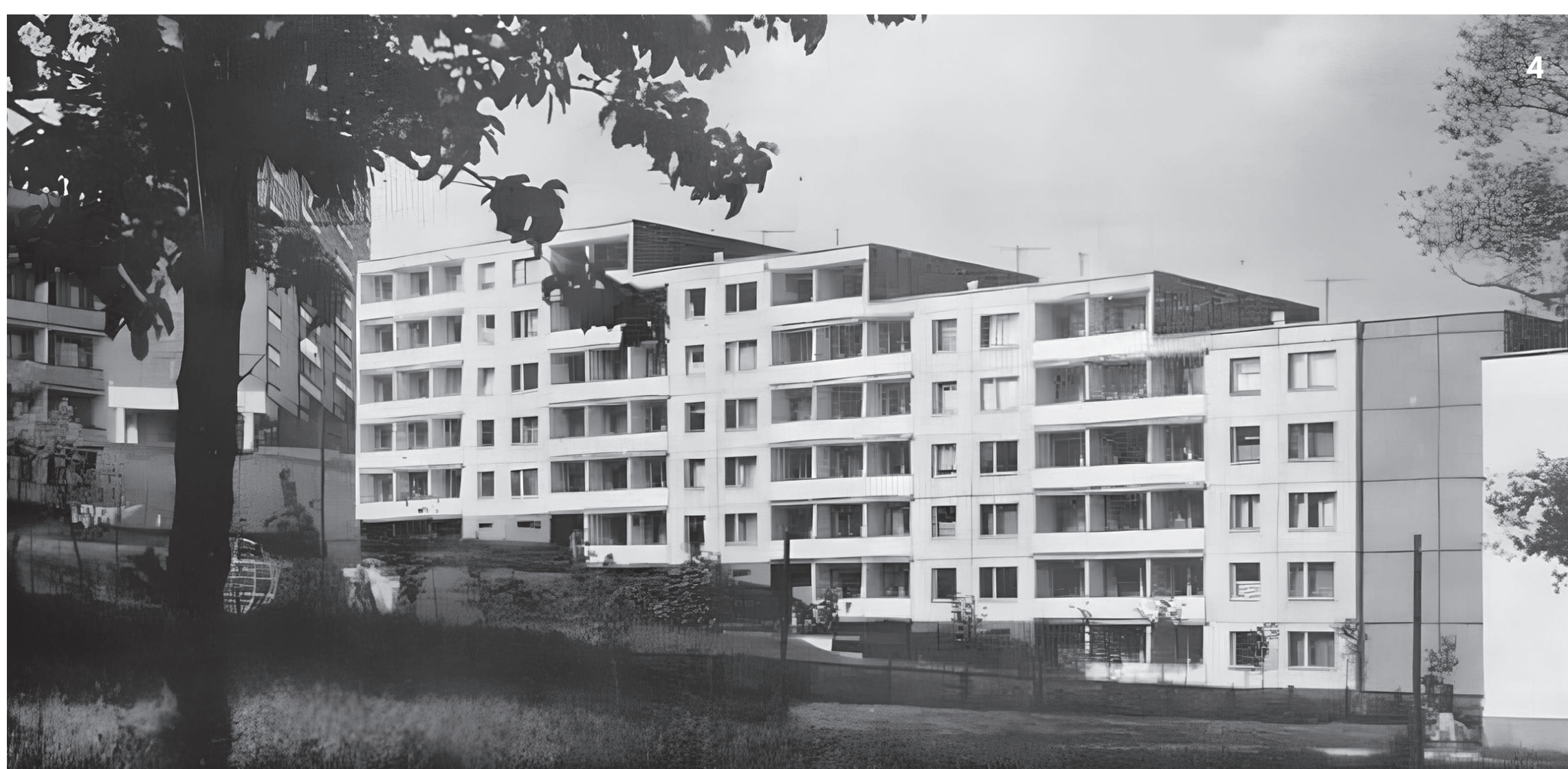
1 Site plan, 2023 2 Initial project, 1967 3 Panorama of the Erfurt Public Centre, 1980 4 Detail of building situated on an elevation, 1980 5 Residential building 1-464 LI series, 2023 6 Yard space of building 1-464 LI series, 2023 7 Tower building, 2023
